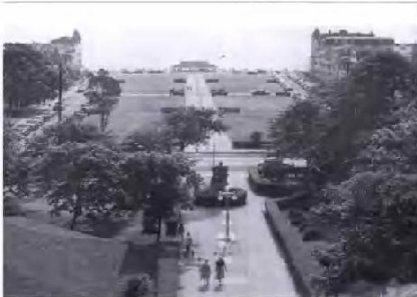
The view from atop the main Auditorium tower, looking east toward the ocean, provides a wide view of Ocean Parkway. Both sides are flanked by large hotels with a mix of single-family homes. Ocean Parkway is one of the most photographed streets by visitors. The Rev. E.H. Stokes monument in front of the Great Auditorium was dedicated on July 31, 1905. Paul W. Murray, a sculptor, cast a bronze heroic-sized form of Reverend Stokes sitting in a chair looking east toward the sea. Participants at the unveiling included New Jersey governor E.C. Stokes, a distant cousin, Bishop Spellmeyer, and A.H. McEvoy, Esp. of Boston Society of Christian Clergy.
